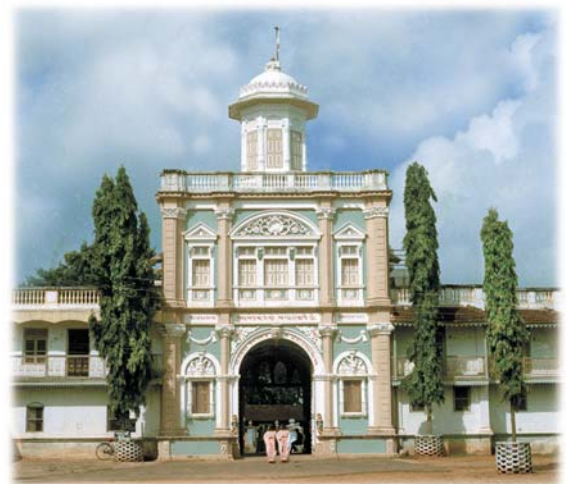
Main Entrance of Ashram
